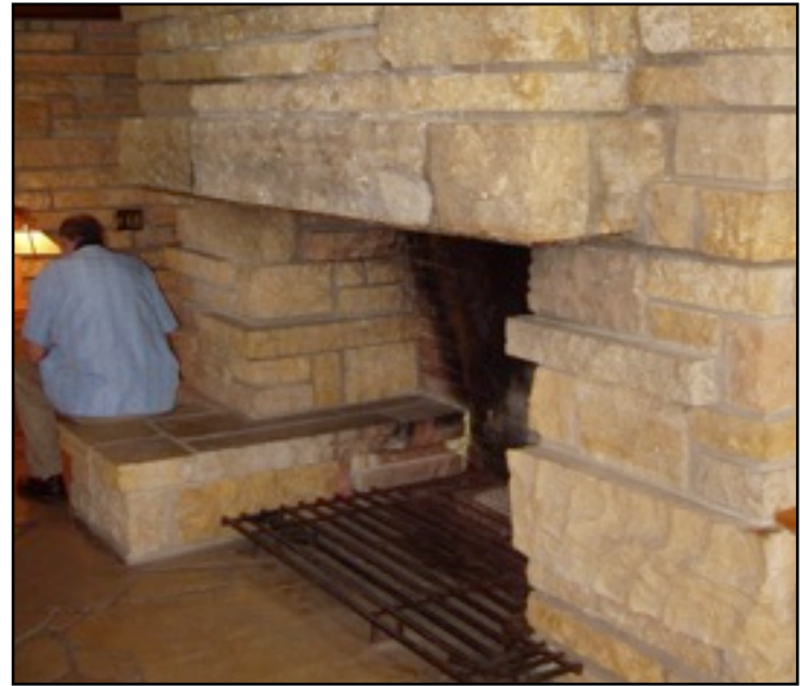
The Lovness Cottage fireplace offers an additional side hearth and features a less-massive, protruding stone hood.
