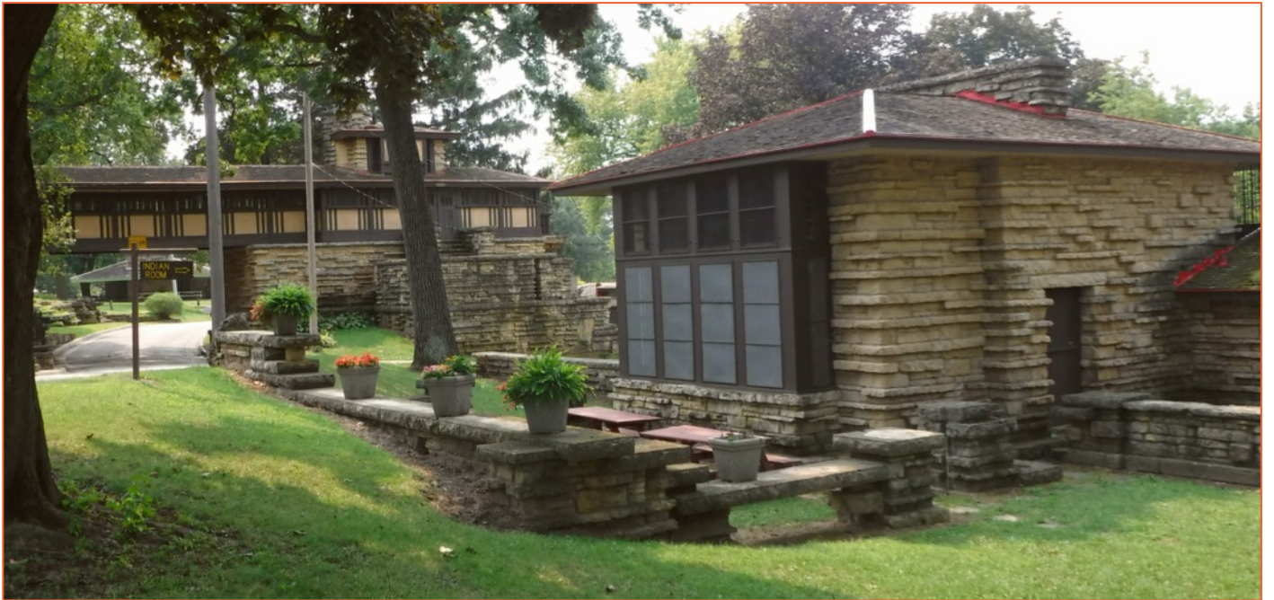
Above: Part of the Bridge Room (left) and Indian Room Buildings (right) Below: Southeast Side of Bridge Complex
