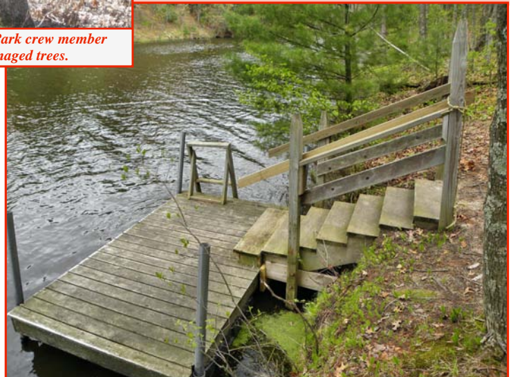
▲ Rebuilt pier steps damaged by last year's flooding.
